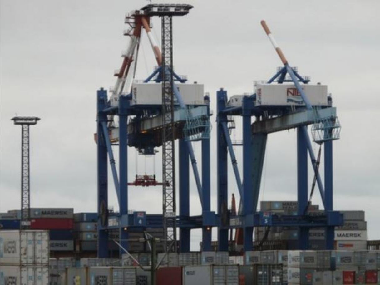
The damaged container bridge in Bremerhaven, Image: Radio Bremen
